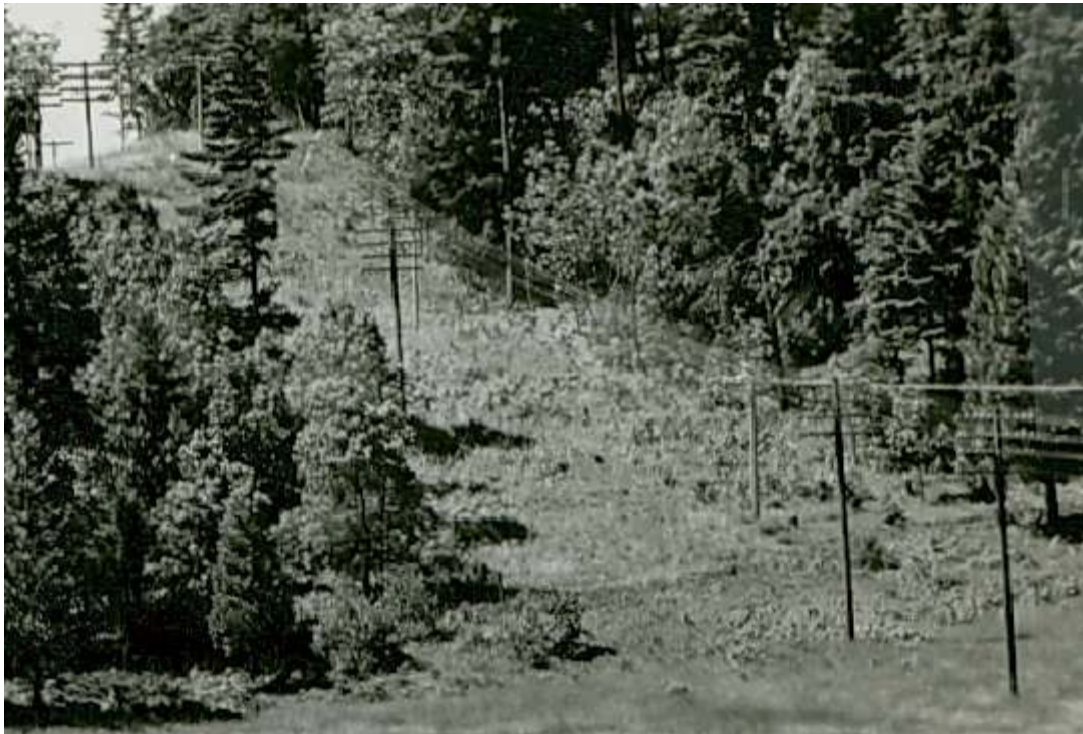
Photo 4B. AT&T & PT Communication Lines Within AT&T 60' ROW In West Field At North Sexton Pass: 1940
