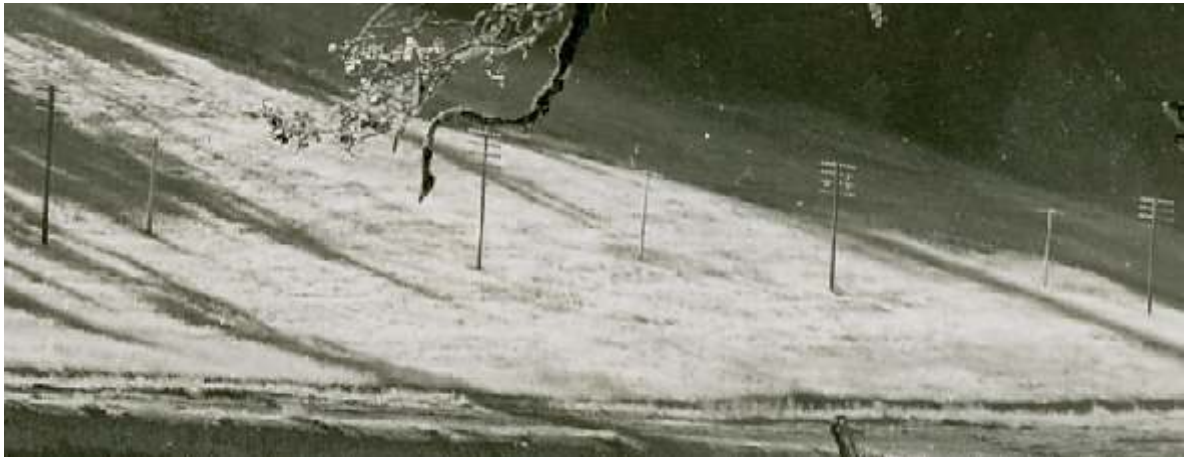
Photo 5B. AT&T & PT Communications Lines In West Field At North Sexton Pass: 1940
