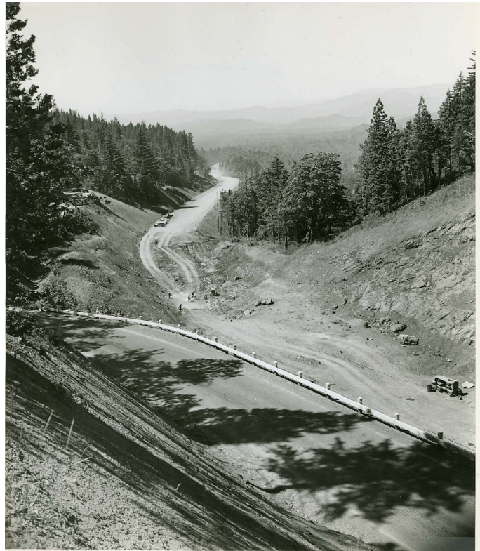
Taking out lower cut thru Summit. Looking S. from S. side of summit cut. Detour in foreground & finish grade in background. Grave Cr.-Jumpoff Joe Cr. Sec., Pac. Hwy. #1845
