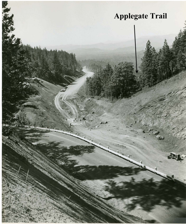
Taking out lower cut thru Summit. Looking S. from S. side of summit cut. Detour in foreground & finish grade in background. Grave Cr.-Jumpoff Joe Cr. Sec., Pac. Hwy. #1845
