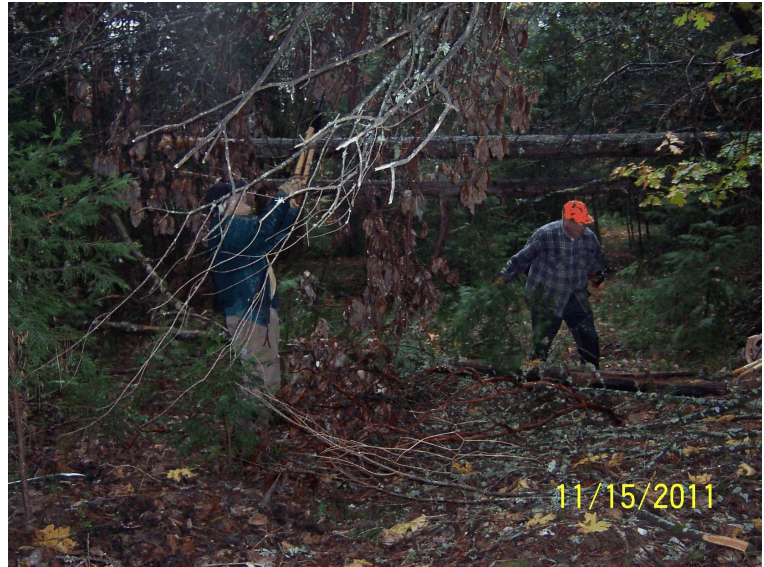
Photo 5. Joe & Jim Brushing At Station 7+60
