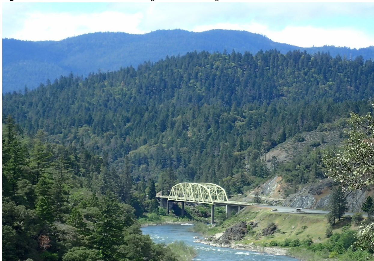
Figure 10.3-10 Photo from KOP #8 looking northwest – Hellgate Overlook
