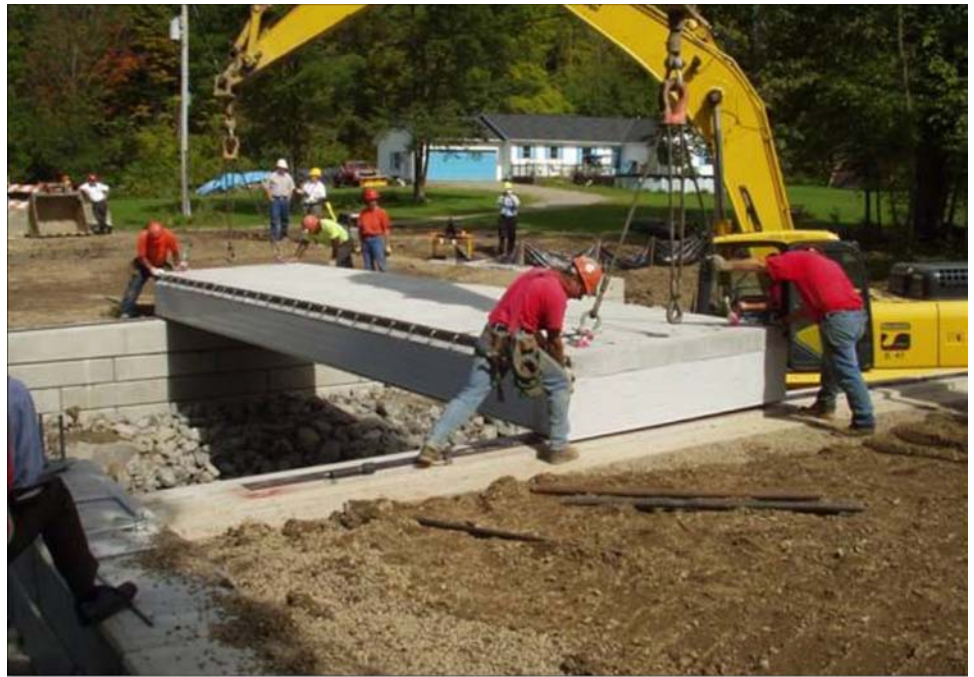
Figure 3: Prefabricated Bridge Elements at Construction Site
