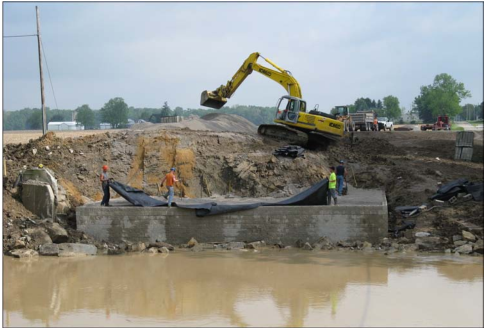
Figure 4: Geosynthetic Reinforced Soil Technology at a Bridge Construction Site
