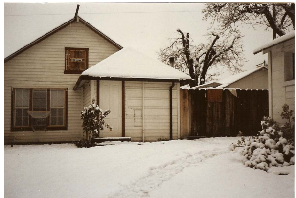
Photo 10. West Side/Backyard of Antlers Home
