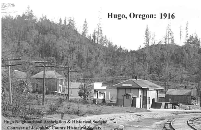
Photo 6. Southern Pacific Railroad's Communications Line
