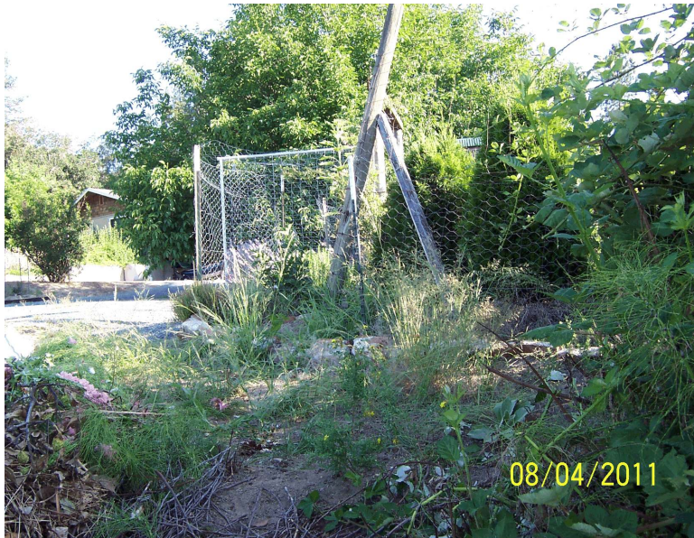
Photo 7. 8' Fence Post At SW Corner of Garden
