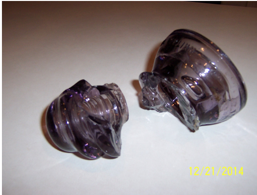
Photo 5a. Broken Garbers Pass Insulator
