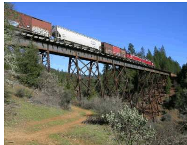
Photo 3. Grave Creek Bridge: 2010
