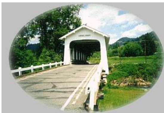
Grave Creek Bridge
