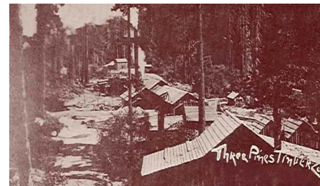
Three Pines Company's Timber Mill At Mountain, Oregon: ca., 1910
