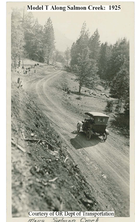
Pacific Highway Along Salmon Creek: 1925
