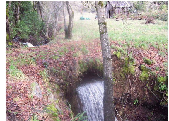
Photo 3. Old Culvert Crossing & Barn: 2006
