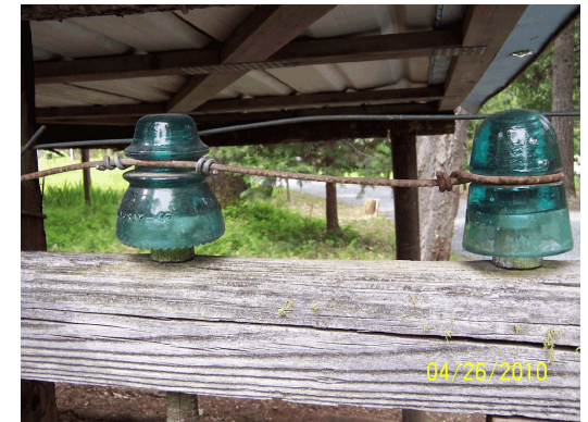
Insulator Line & Insulator Ties
