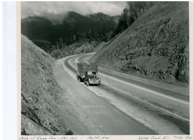
U.S. 99 at Windy Gap on Mt. Sexton: 1951 Courtesy of Oregon Department Of Transportation
