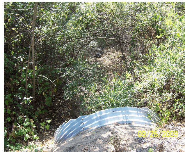
Bannister Creek Culvert Under Hidden Acres Drive
