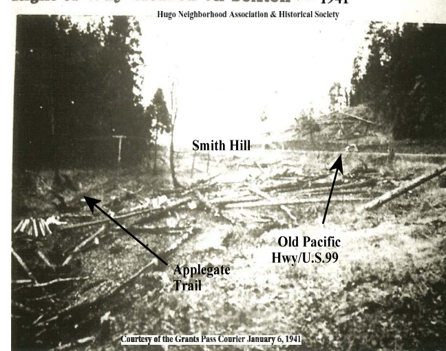
Photo 1. Postal Telegraph Pole Middle Left Photo At Mt. Sexton Pass Before Cut: 1941 Courtesy of the Grants Pass Daily Courier
