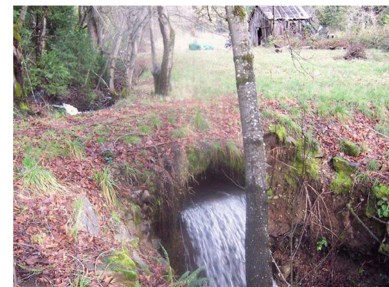
Photo 3. Old Culvert Crossing & Barn: 2006
