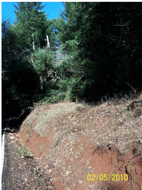
Photo 5. Fiber Cable Route North Of Old Stage Road
