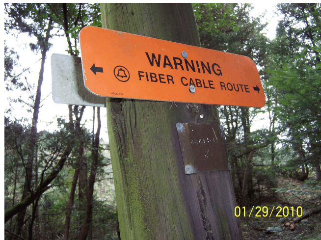
Photo 1. Fiber Cable Route Sign South of JA-15
