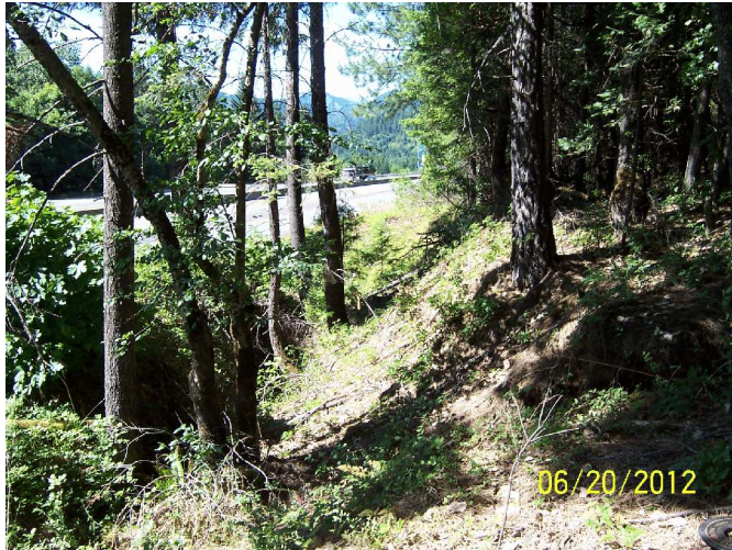
Photo 7. New ODOT Cut-Slope Below Last 150' Of ATI
