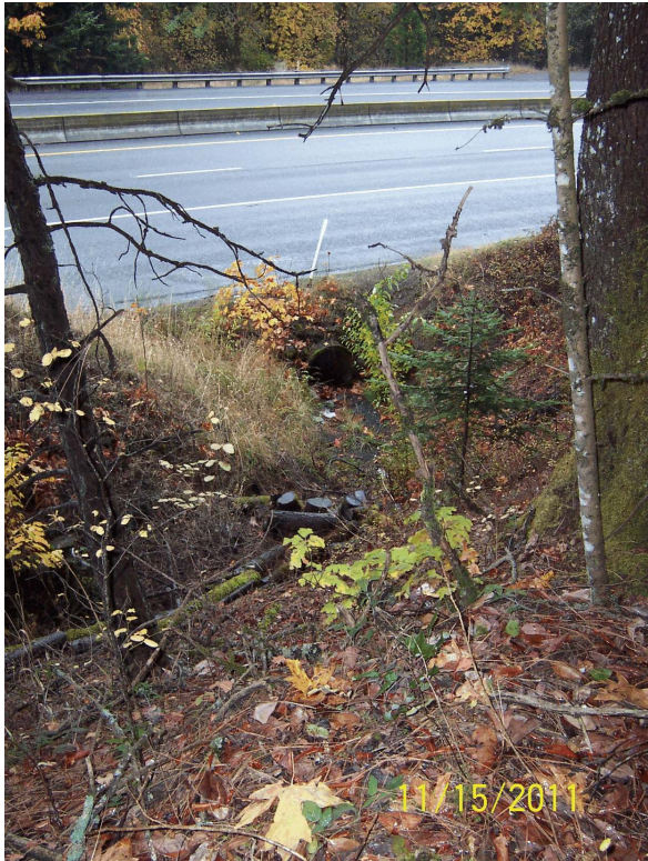
Photo 4. I-5 Culvert At Station ATI 10+00
