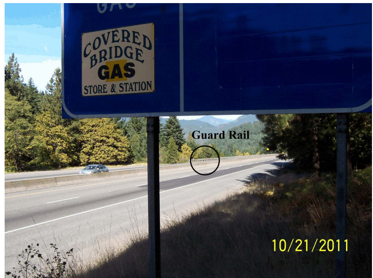
Photo 6. Guard Rail West Toward JA-15 From I-5 Sign
