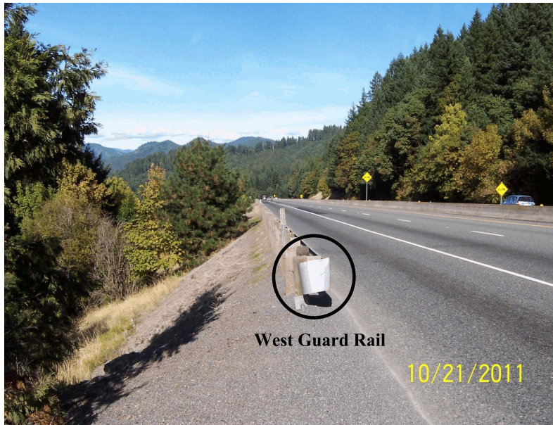
Photo 8. I-5 Guard Rail Along Trail Near JA-15
