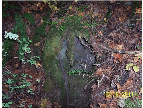
Photo 6. West End Of Culvert
